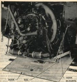
Figure 255—Door Plate Lowered, Giving Access to Bottom of Engine
