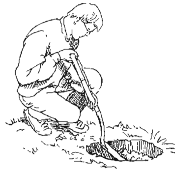
FIGURE 7.2. A proper shoveling stance keeps your back straight at all times and uses your legs, your arms, and the levering action of the shovel to do the work. When working in a deep hole or with a D-handled shovel, squatting is the best position, as shown here. Long-handled shovels should be used when standing fully upright.
