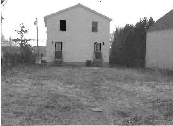
FIGURE 3.14. Looking southeast from the far end of Eric Toensmeier's and Jonathan Bates's backyard in Holyoke, Massachusetts. This site, our design-process case study, has a new duplex that was built after the previous home burned down. Clearly, this site needs healing attention. The barn and arborvitae hedge to the south (right) are owned by the neighbor.
