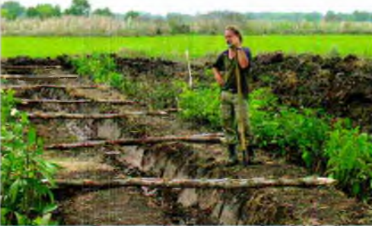
My colleague of many years Erich Auernig prepares a canopy for the trench.
