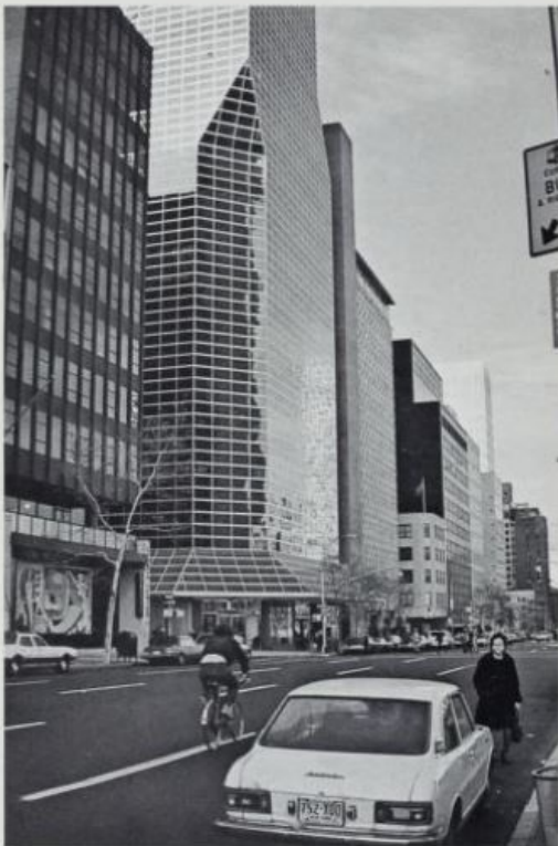
642. Kevin Roche and John Dinkeloo, United Nations Development Corporation, begun in 1969, New York
