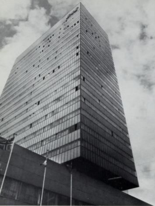
599. Arne Jacobsen, SAS Building, Copenhagen, 1957-62 600. Riccardo Morandi, viaduct, over the Torrente Polcevera, Genoa, 1967
