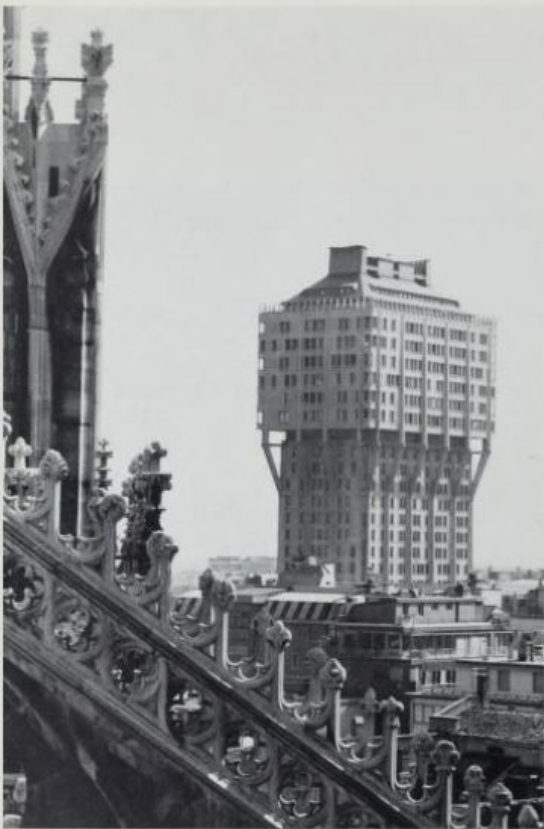
622. BPR (L. Belgiojoso, E. Perissutti, E. Rogers), Torre Velasca seen from the Duomo, Milan, 1956-58
